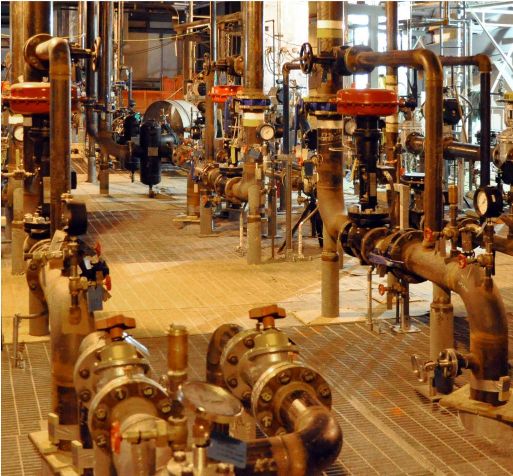
Kurz 534FTB inline flow meters for industrial gas flow measurement are designed to eliminate the need for field fabrication and assembly of inlet and outlet piping sizes by providing accurate gas flow measurement under changing upstream and downstream flow profiles. Built-in reducers/expanders result in exceptional immunity to upstream and downstream flow disturbances caused by valves, bends, and short straight runs.
